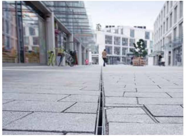
Surface drainage with tailor-made slotted channels.
